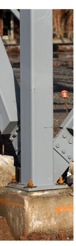
Figure 1 – Steelwork Fire Protected by SFRM Coating System Photo courtesy of GCP Applied Technologies
