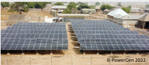
PV array on a recently commissioned PowerGen microgrid in Nigeria. Project photos and software screen captures courtesy of PowerGen
